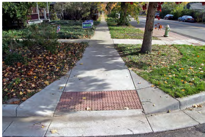
Ramps with textured surfaces help make streets accessible for all users. Photo credit: www.pedbikeimages.org /Dan Burden
