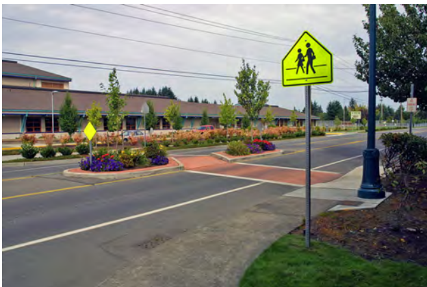
Pedestrian refuge islands break up wide street crossings.
